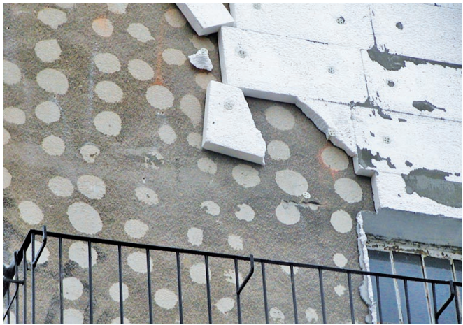
Careless preparation of the substrate and above all not cleaning of dirt or grease and not removing old coatings, results, in most cases, in disruption of the thermal insulation of the entire wall surface. In the pictures are shown errors and their consequences.
