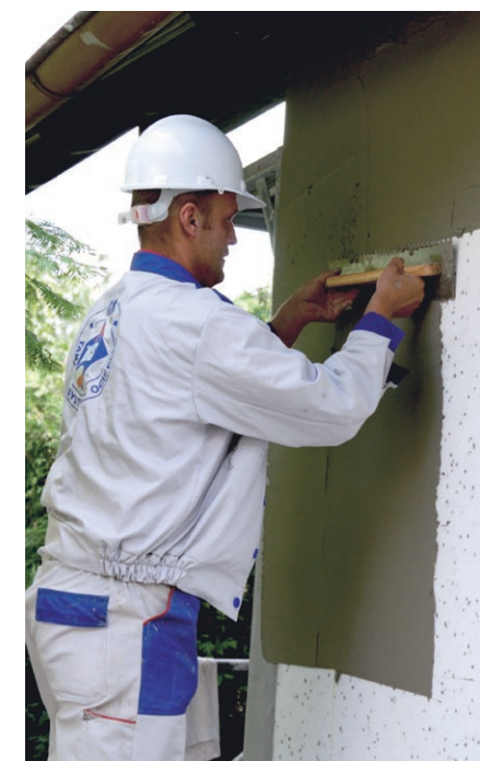
APPLICATION OF ADHESIVE ON POLYSTYRENE
