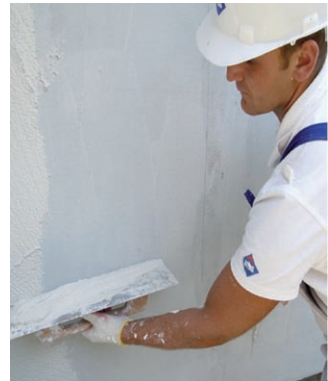
Applying renders using steel trowel
