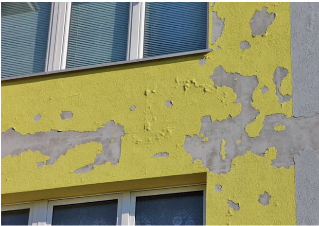
Careless preparation of the substrate and above all not cleaning of dirt or grease and not removing old coatings, results, in most cases, in disruption of the thermal insulation of the entire wall surface. In the pictures are shown errors and their consequences.
