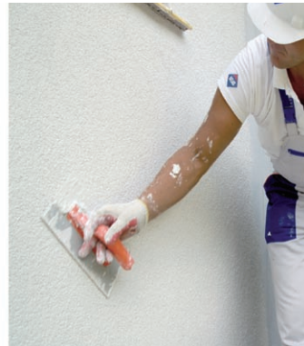
Applying renders using steel trowel
